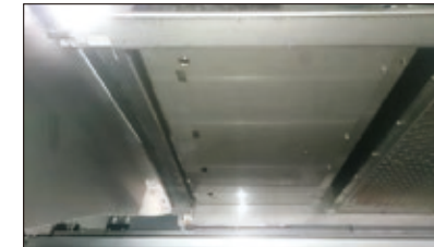
清掃直後 After cleaning
